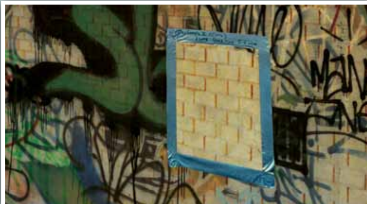
Graffiti is easily removed from the protected surface
