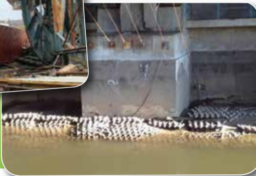
A-Jacks® provided bridge pier foundation scour protection to withstand Hurricane Sandy.
